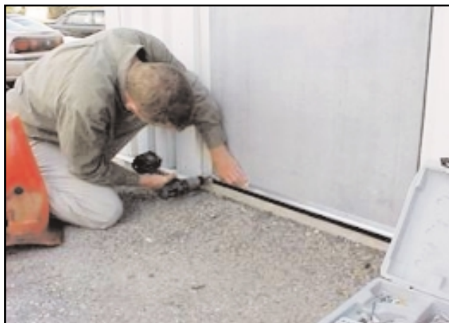
Keep Out: An Integrated Pest Management program includes common-sense practices such as sealing openings, cracks, and crevices.
