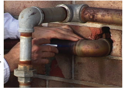
Inspect the exterior of your building for pest entry points such as utility penetrations.
