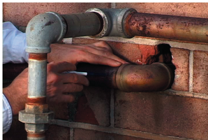
Figure 3. The places where utility services penetrate the façade of the building provide a perfect entrance for pests. Be sure to inspect the exterior of your facility with a pest management provider and your onsite maintenance team to identify locations that need sealing or repairs to prevent pests from slipping inside.
