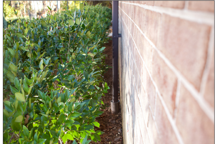
Trimming back vegetation at least 2 feet from a building deters pests from getting inside.
