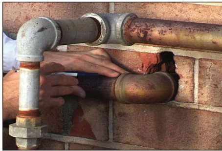
To prevent pest infiltration, identify and seal unnecessary openings in the facility's exterior wall with a water-resistant sealant.
