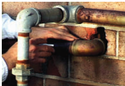
Since a rodent can enter a building through an opening the size of a pencil, seal all unnecessary openings with weather-resistant sealant.
